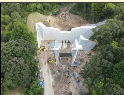
(10) 2021.9 帯工(Co打設)
