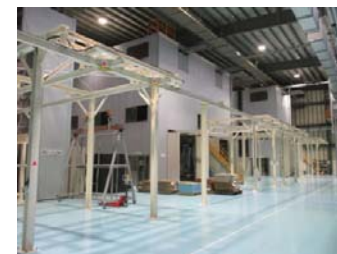
Sulfuric Acid Anodizing Line
