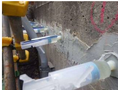
躯体ひび割れ補修
