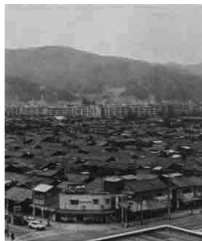
Photo5-a Wooden public housing in the Moto-machi district (Collection of Housing Policy Division, Urban Development Bureau, the City of Hiroshima)
