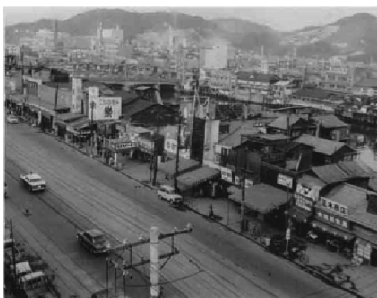
Photo 5-3 Illegal postwar riverbank construction cluster in the Matoba district near Hiroshima Station. (Courtesy of Hiroshima Municipal Archives)
