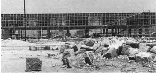
The display hall under construction (July 1, 1952) (Courtesy of Hiroshima Municipal Archives)
