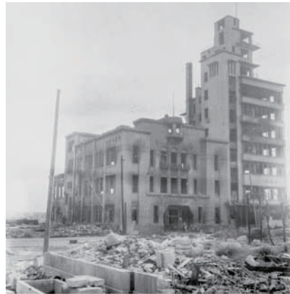
The Chugoku Shimbun's head office building after being completely destroyed by the fires of the atomic bombing in 1945. (Photo by Toshio Kawamoto, Collection of Hiroshima Peace Memorial Museum)
