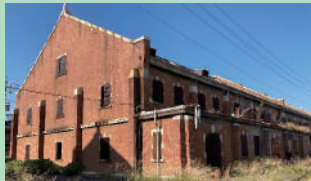
Former Army Clothing Depot
