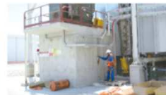
Plant test operation
