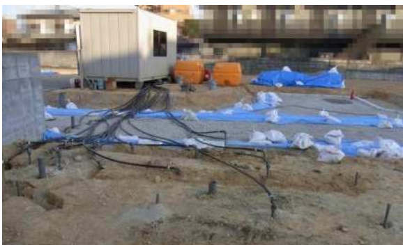
In-situ injection of reactants
